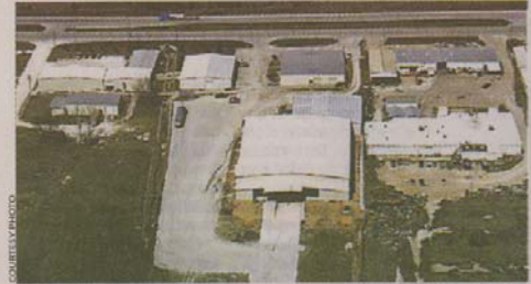
MOLDING THE FUTURE: K&D Plastics Inc. operates from a manufacturing plant in Gainesville, supplying components to the commercial aircraft industry.
